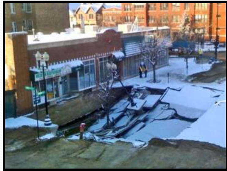
Main break in Ravenswood - photo MSNBC
